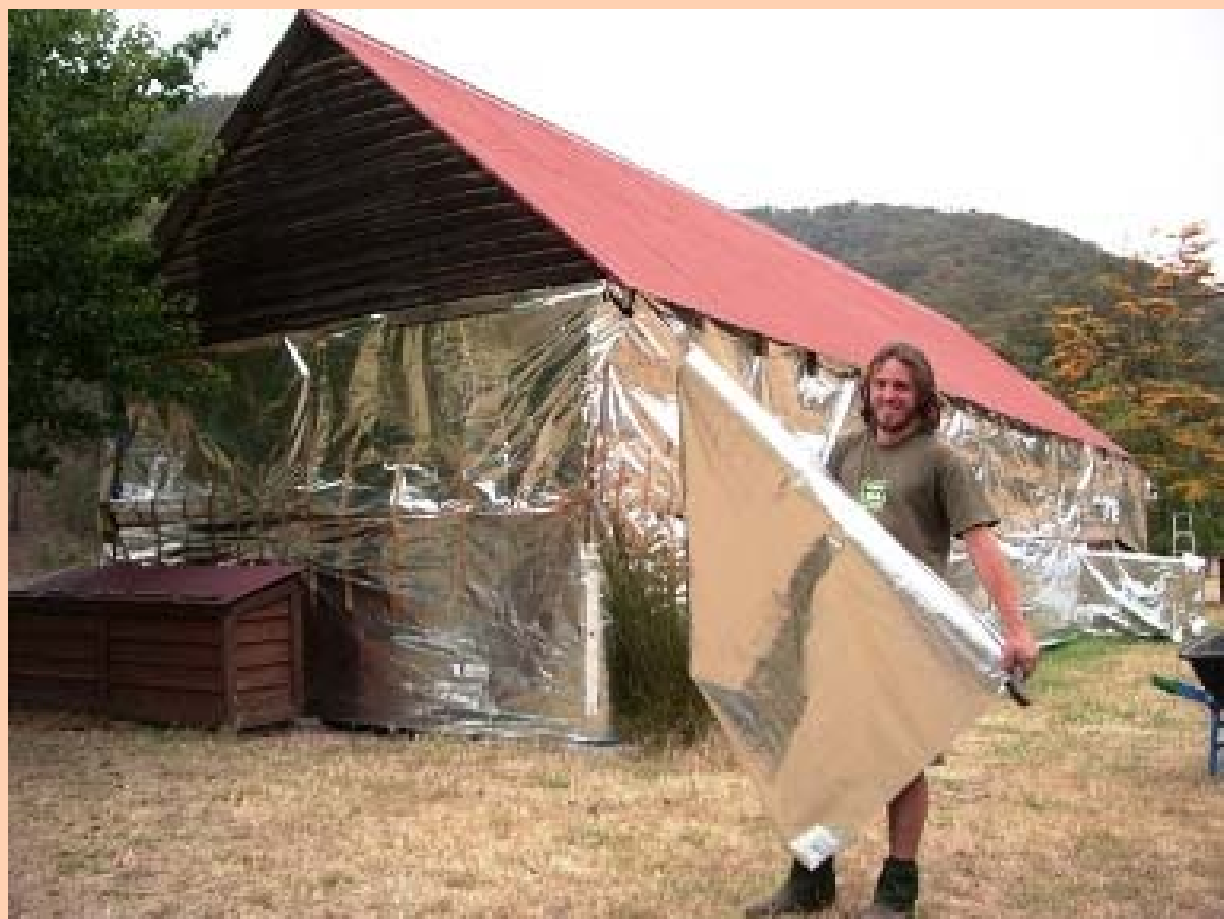
Wrapping in foil at Wollangarra (not a hut) prior to the 2006-07 fires.
