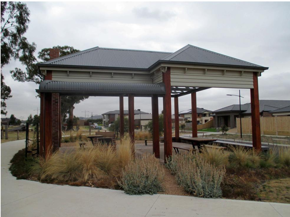
Heritage farmhouse interpretative shelter at Epping North, City of Whittlesea. In this new housing estate the shell of a heritage place provides a barbecue and an interpretative panel. The frame of the house has been completely replaced with a steel structure. (Source: Context 2014)
