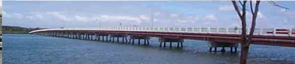
Bribie Island Bridge 1963
