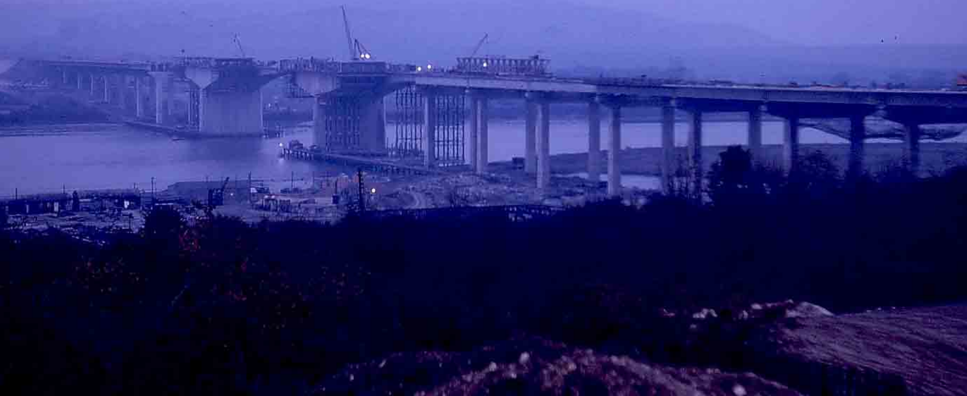
Ulrich Finsterwalder/G Lohmer Bendorf Bridge , Koblenz 1960-65 Freeman Fox Medway Bridge on M2, Kent under construction (completed 1960)
