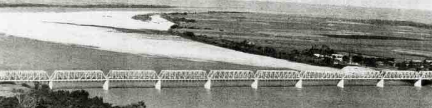
Burdekin Bridge (COG Report 1958, QPP)
