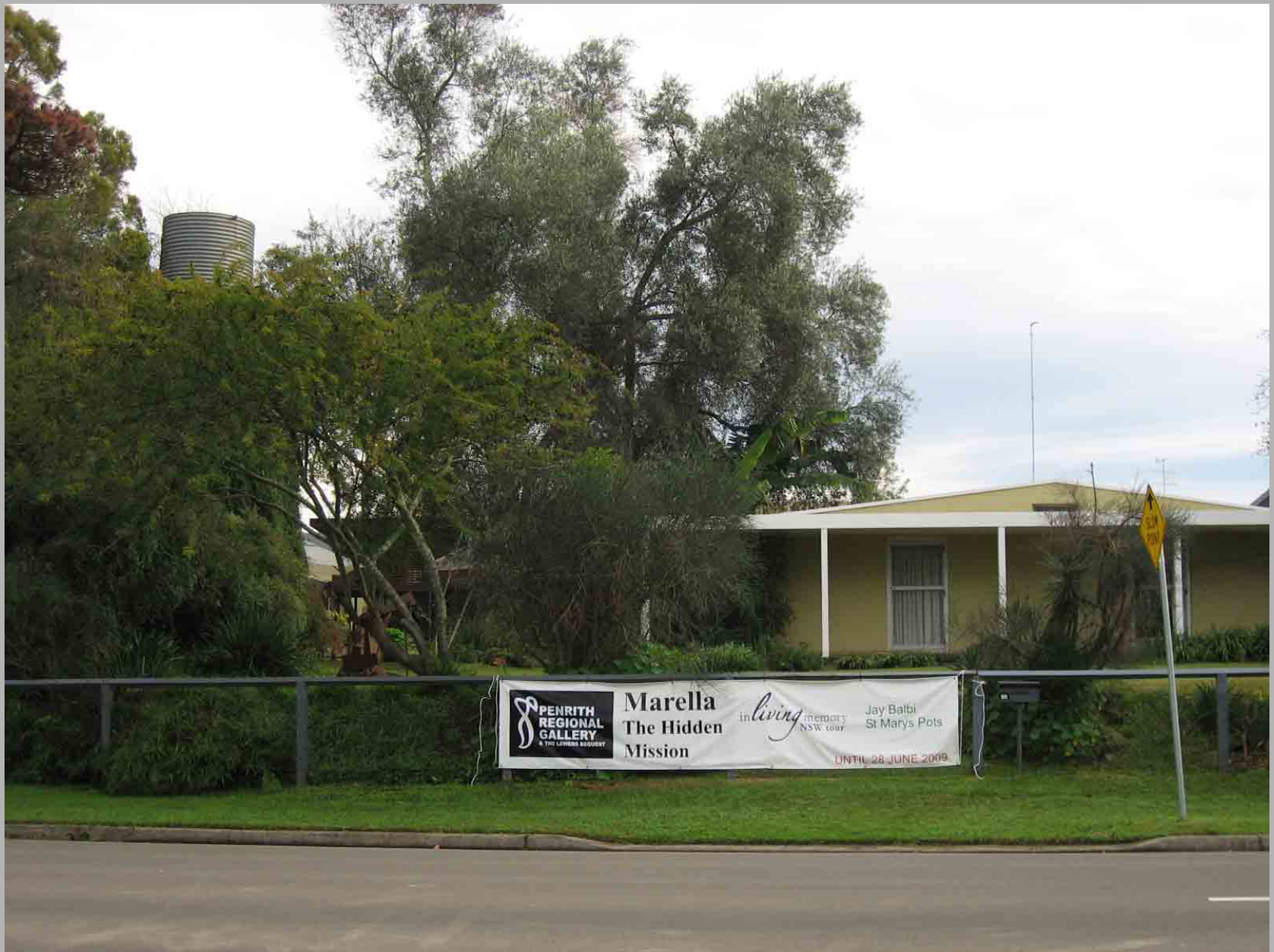
Ancher house, constructed 1961-64
