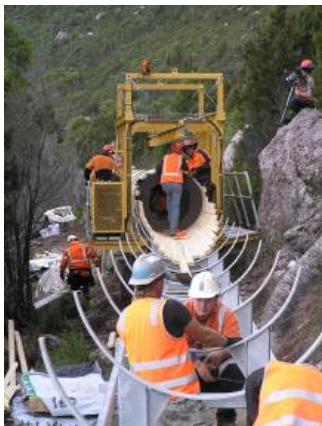
Constructing the new woodstave pipeline in April 2009
