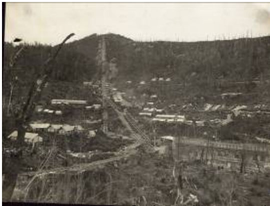
Lake Margaret Power Station under construction
