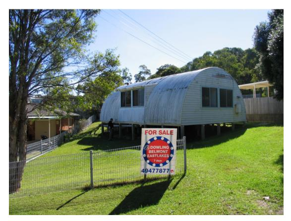
The Nissen hut purchased by the HHT is a 3 bedroom; 24' span DB3 type. The building is in a 'tired' condition and is perched on concrete stumps on a difficult sloping triangular block. Not surprisingly the HHT was the only party interested in purchasing the hut.
