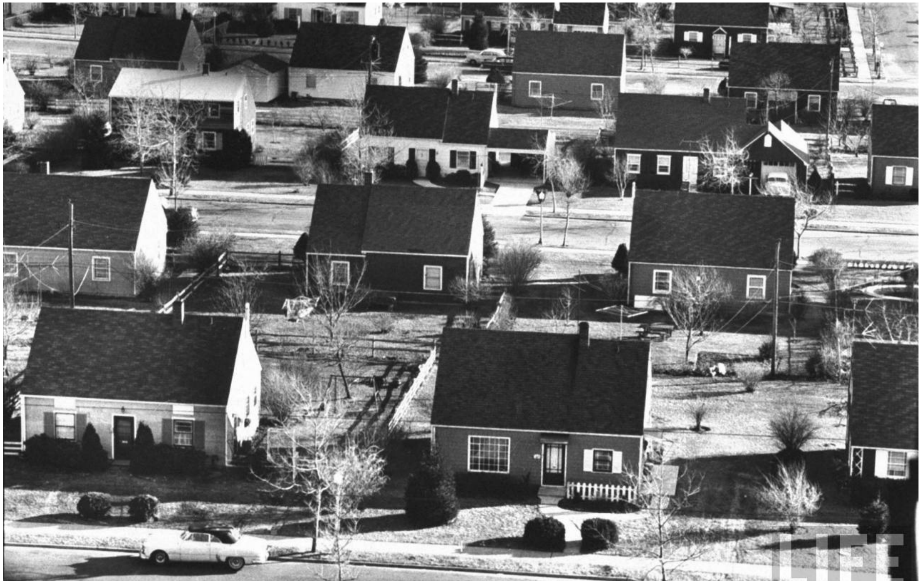
Levittown, Long Island, NY, 1947-1951 - Levitt & Sons, Inc
