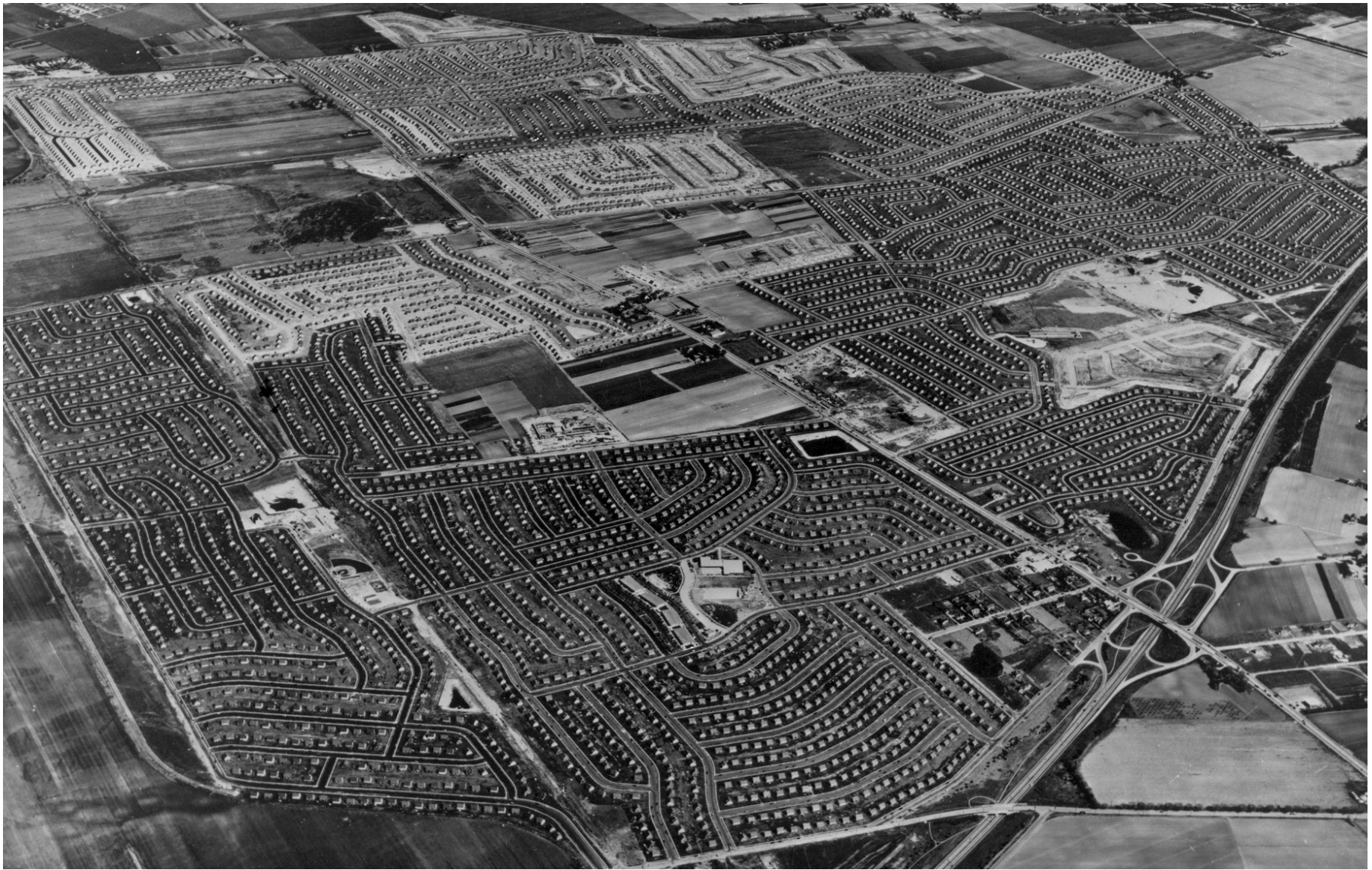
Levittown, Long Island, NY, 1947-1951 - Levitt & Sons, Inc
