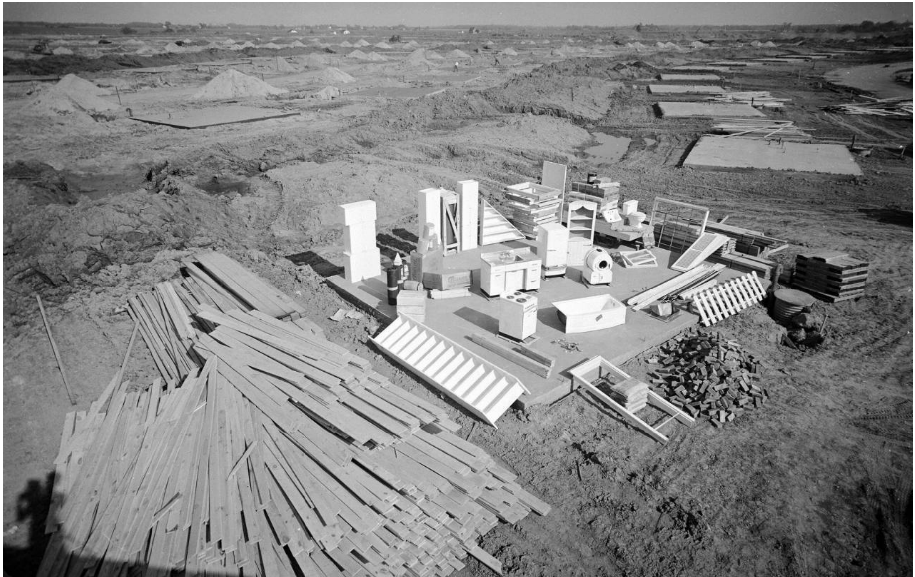
Levittown, Long Island, NY, 1947-1951 - Levitt & Sons, Inc
