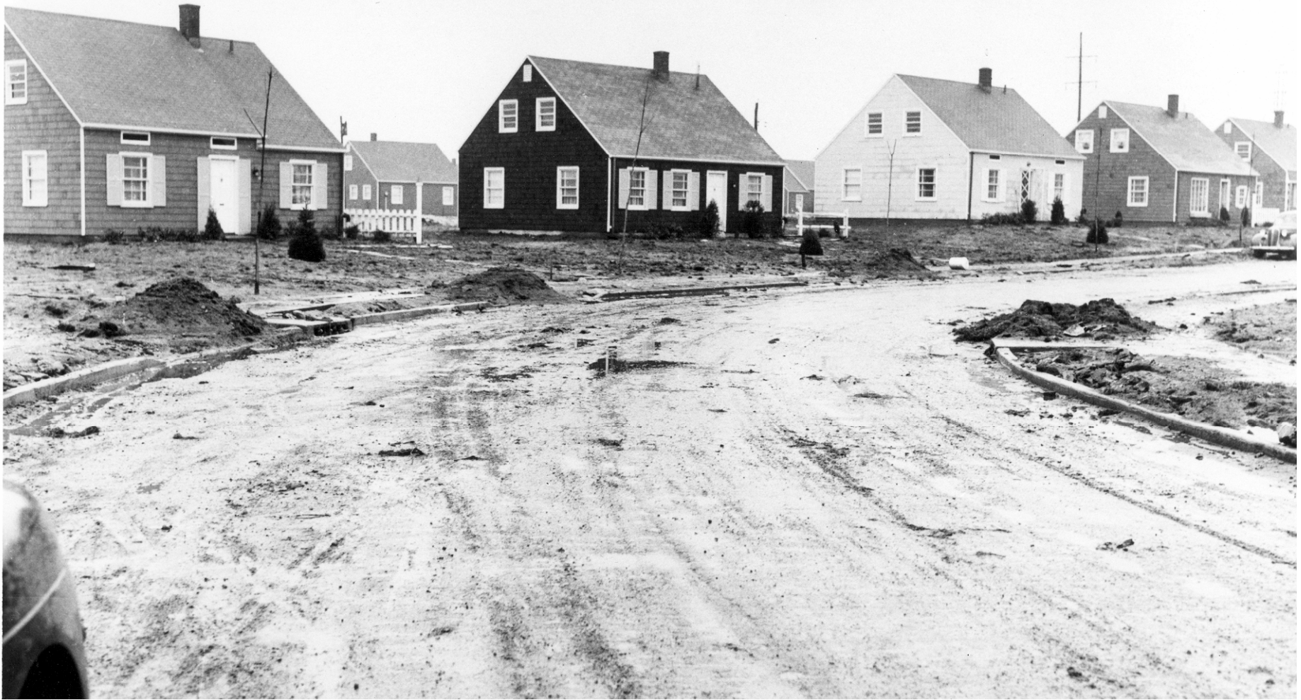
Levittown, Long Island, NY, 1947-1951 - Levitt & Sons, Inc
