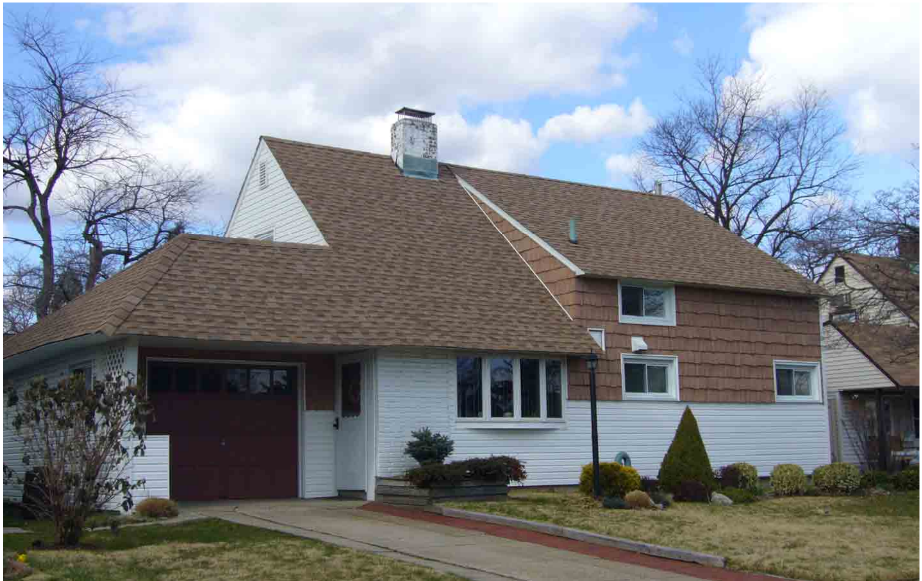
Levittown, Long Island, NY, 1947-1951 - Levitt & Sons, Inc
