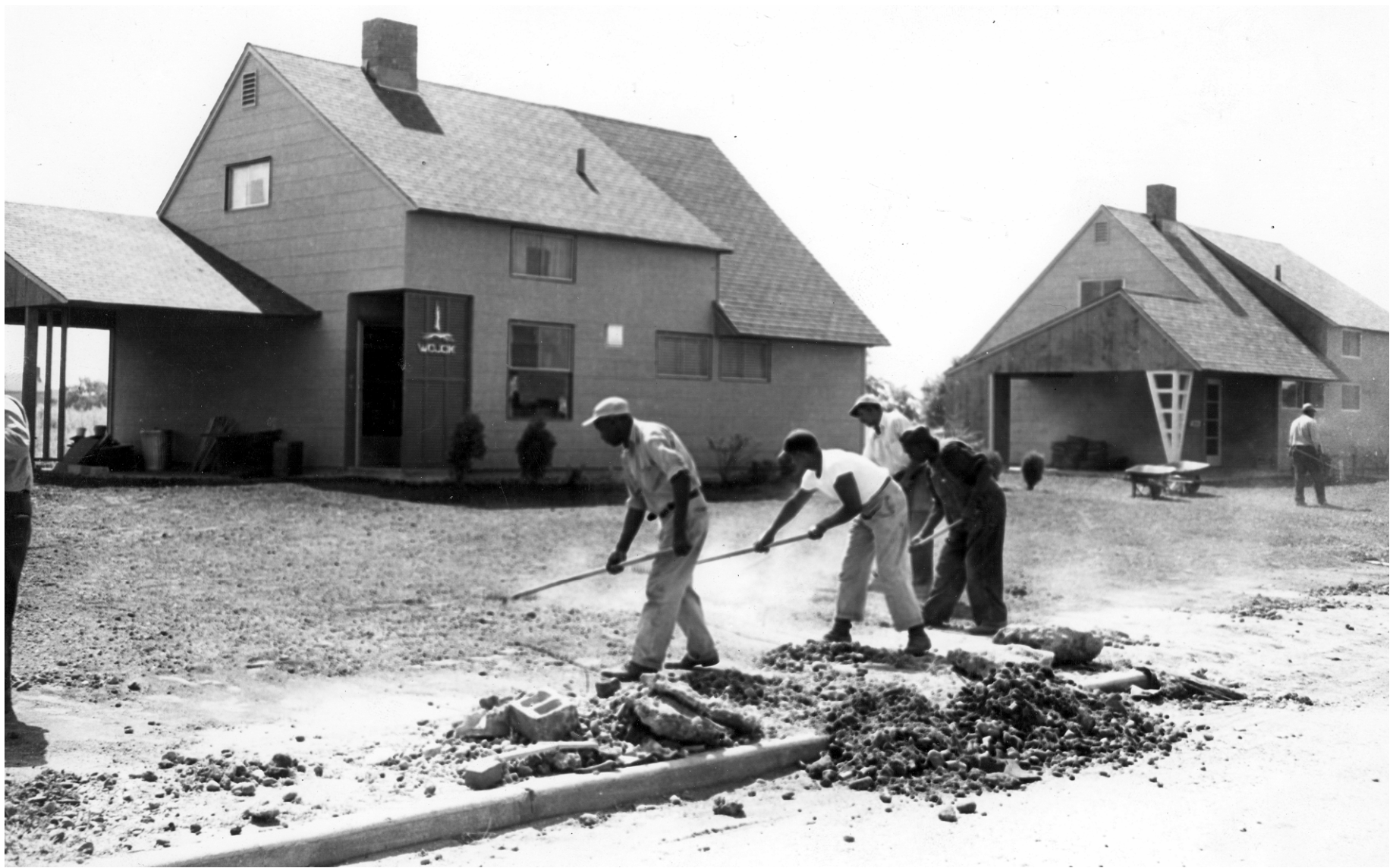
Levittown, Long Island, NY, 1947-1951 - Levitt & Sons, Inc
