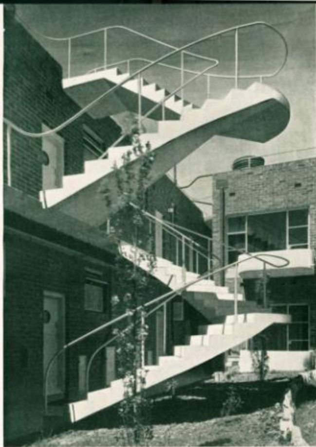
The Outside Staircase, with its metal banister and concrete steps is strikingly modernistic.
