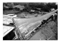
FIG 19 hyperbolic/parabolic roof under construction.
