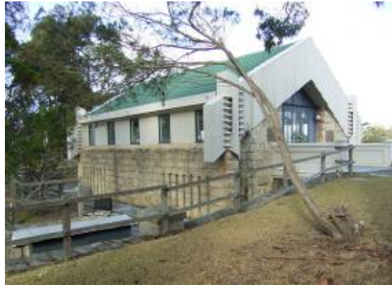
Figure 3: Incinerator in July 2004 View on the delivery floor from north-west.
