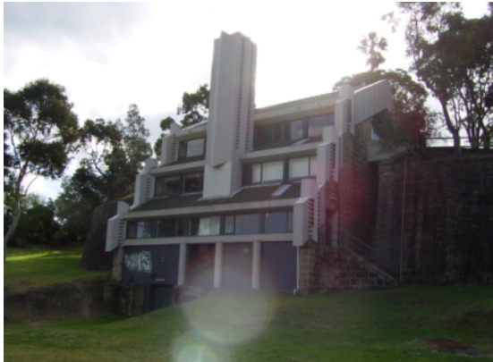
Figure 2: Incinerator in July 2004 View from south-east. Delivery floor at the top, trimmer's floor, furnace floor and ash floor below.
