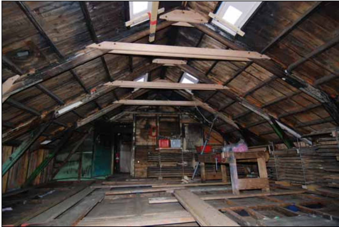
Figure 3: Biscoe Hut, Mawson station during repairs (Mike Staples, 2007: © AAD)
