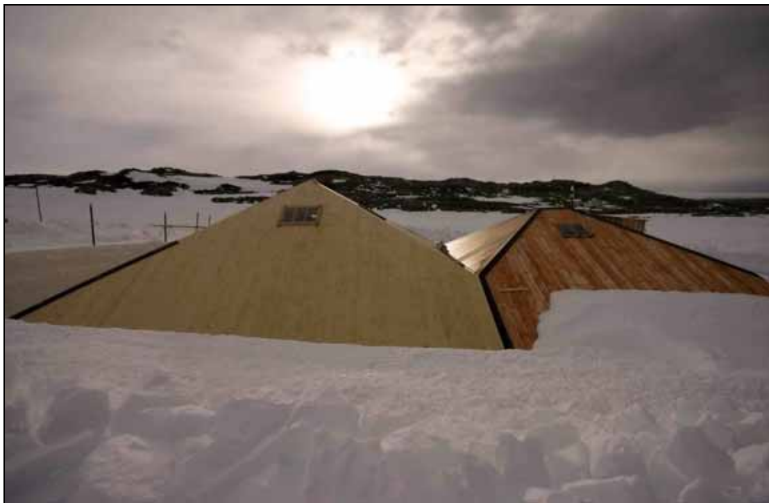
Figure 2: The Main Hut, after over-cladding (Simon Mossmann, 2006: Mawson's Huts Foundation, AAD collection)
