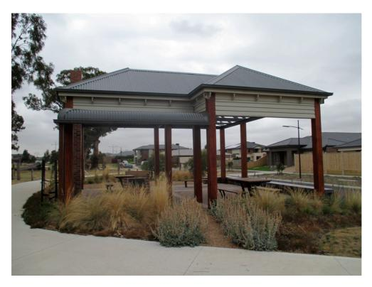
Heritage farmhouse interpretative shelter at Epping North, City of Whittlesea. In this new housing estate the shell of a heritage place provides a barbecue and an interpretative panel. The frame of the house has been completely replaced with a steel structure. (Source: Context 2014)
