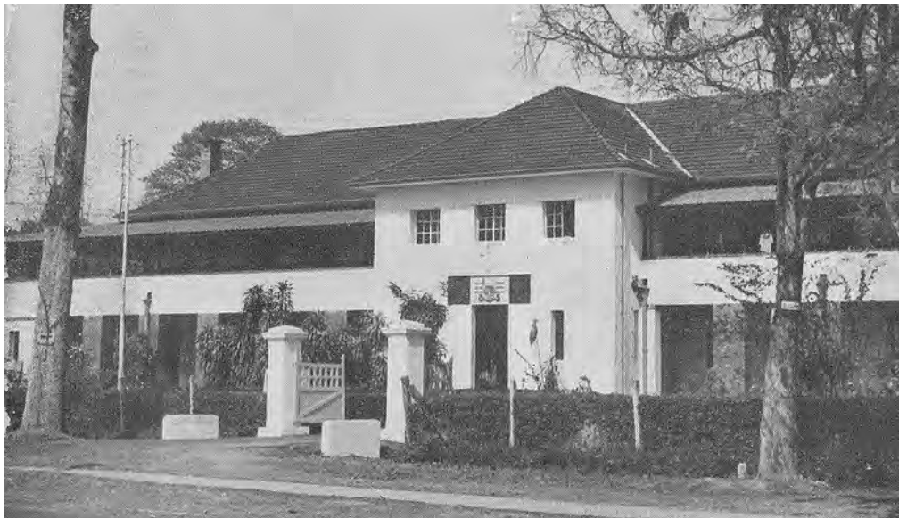
Figure 3 View of the student union building from Chancellor Road Drive: only the gate posts survive Source: Accessed online via Google Images, 7 September 2015
