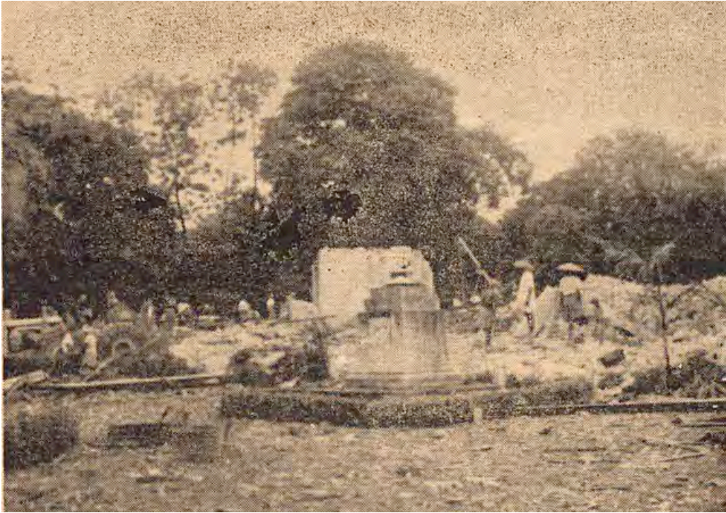
Figure 4 The Student Union building following demolition, 7 or 8 July 1962 Source: Mizzima, Photo Essay, 'Historical Photographs July 7, 1962', http://archive-2.mizzima.com/gallery , accessed 7 September 2015
