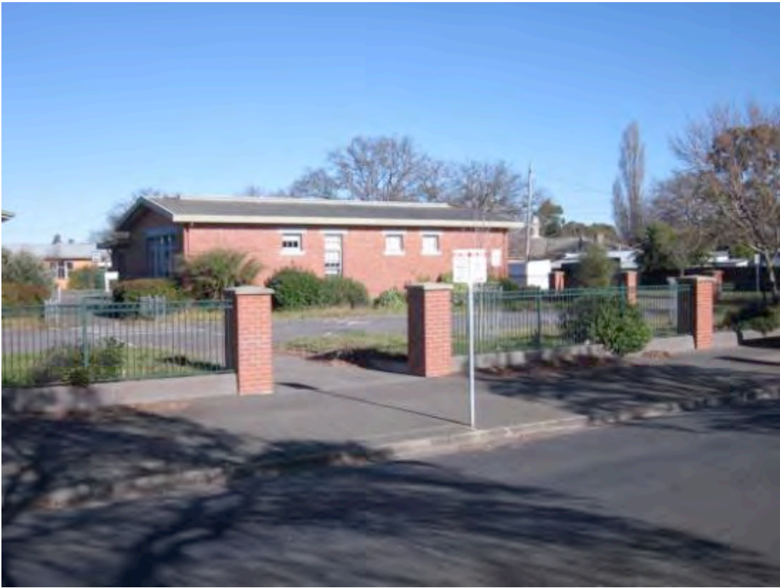
Figure 3 View of the 1919 Schoolhouse from Victoria Street (Lovell Chen, 2011)
