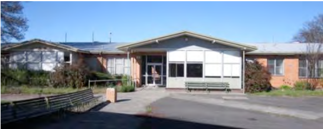
Figure 4 The Albert Leach Cottage wing constructed 1964 (Lovell Chen, 2011)
