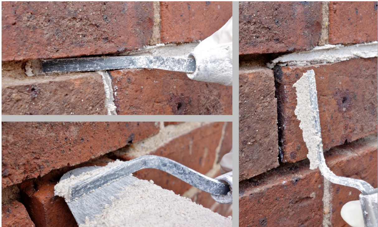
Figure 6 Placing mortar with trowels that fit within the joints means that no mortar need be smeared on the face of the brickwork, and no acid clean-up is required.
