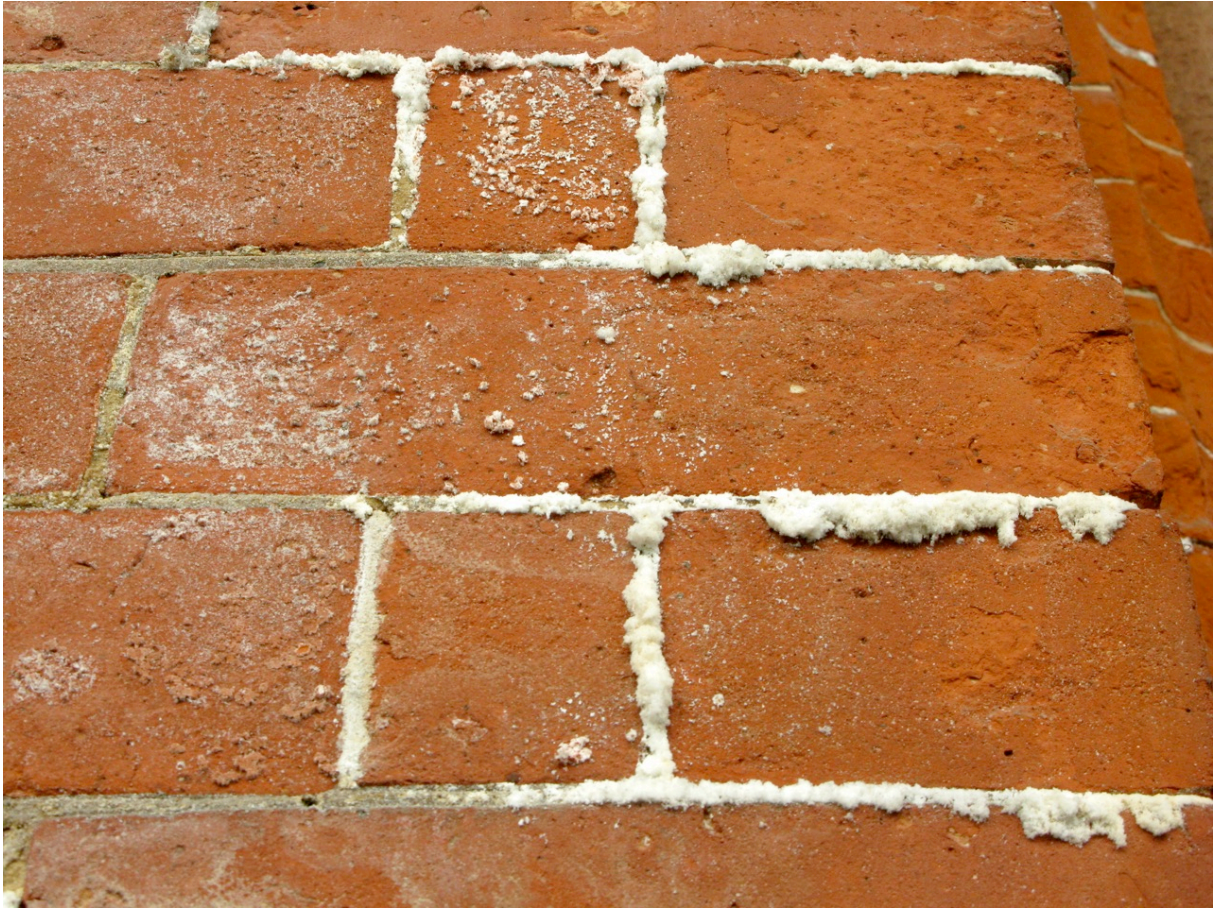
Figure 1 Permeable mortar allows moisture transport and evaporation through the joints, here graphically illustrated by salt crystallising at the surface.
