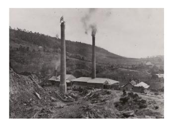
Two Hoffman style kilns were built at the Knocklofty site on the hills of Hobart. Here the second kiln is under construction in about 1913 under the ownership of Crisp and Gunn. Plans were floated for a third kiln, but it was never realised.
