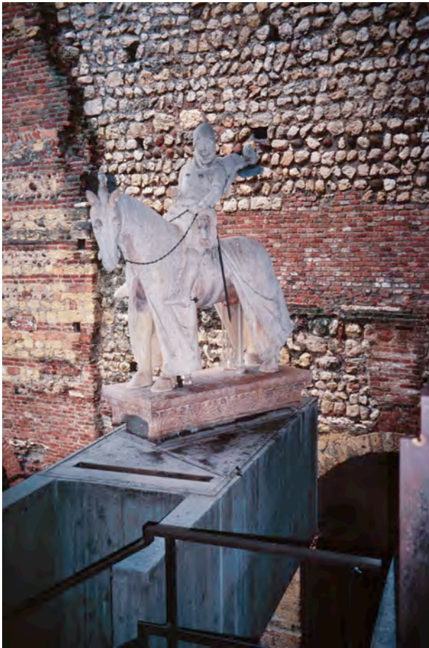
Modern insertions by the architect Carlo Scarpa that serve to also reveal historic phases of use, Castelvecchio, Verona. Photo by the author
