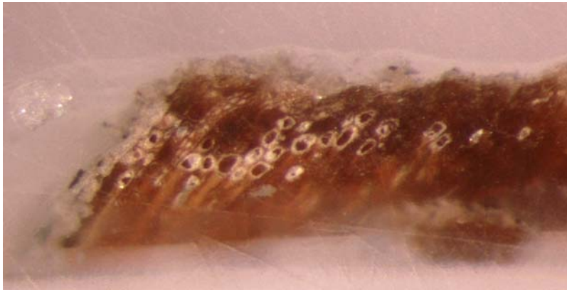
Figure 4. Microphotograph (40x) of a sample taken from the outer face of the balcony door (east elevation of front wing). The large brown object is the timber, with a very thin coating of grey paint on its upper and left-hand edge. (N Schmeder, 2014)
