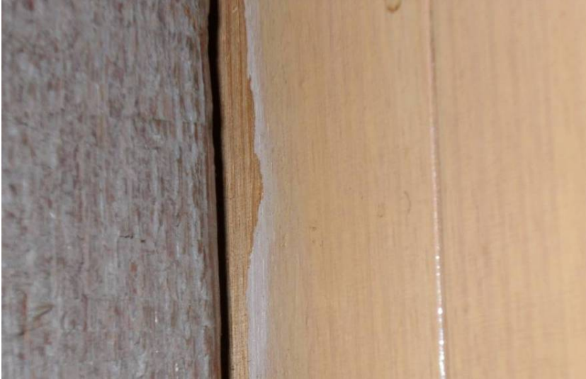
Figure 1. Left to right: Rough-sawn Oregon post with silver-grey coating; ash joinery with unfinished strip, edge of limed finish showing white undercoat, and with varnished top coat (N Schmeder, 2014).
