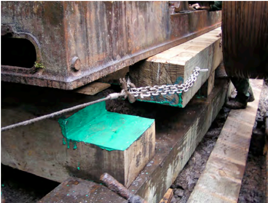
Figure 4: Big River sawmill engine foundation replacement, use of bridge spikes and chain with hand winch to slide beams into position. Note the Koppers CN Emulsion colour. 2006 (Jim Staton)
