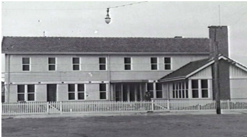
Gordon Street Footscray, War Workers Housing Trust dormitory for Women War Workers, completed in June 1942 and proclaimed as being the first of its type. Source AWM photographic collection v .
