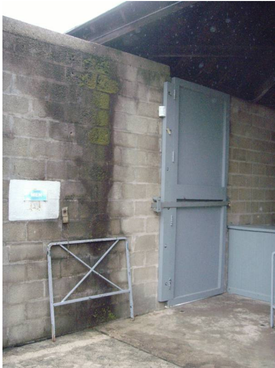
Figure 3: Walls are covered with organic matter where roof run-off occurs.
