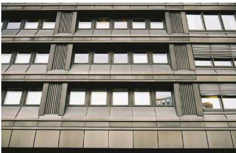
Anodized aluminium became a common façade material in the 1970s. The Gallerian shopping mall block was clad in aluminium sheet metal. The design of the portion facing the Brunkebergstorg square alludes to classical prototypes, hinting at pillars between the windows.
