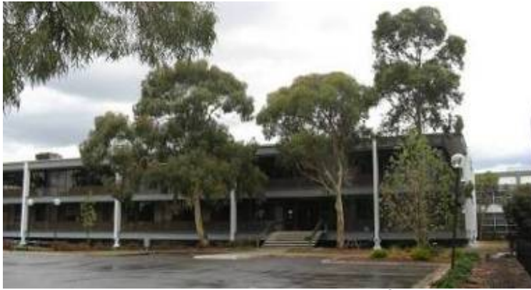
The 1969 building, Eggleston MacDonald and Secomb
