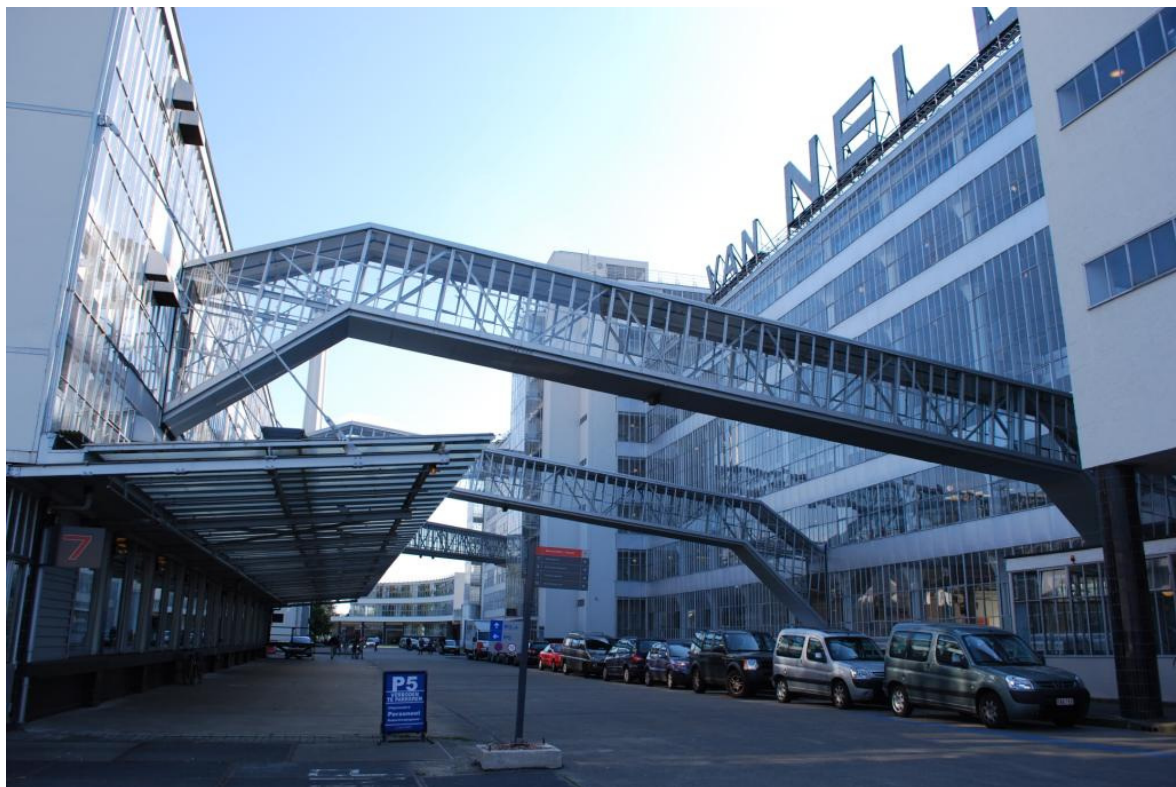
Figure 1: The Van Nelle Factory in Rotterdam (1926-29) designed by Johannes Brinkman with L.C van der Vlugt and Mart Stam. The characteristic curtain wall is of primary importance to the building, both technologically, architecturally and aesthetically.
