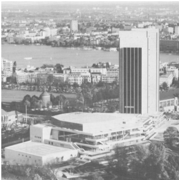
9. The Congress Centre in Hamburg (1970-73) by Jost Schramm and Gerd Pempelfort as a representative of a typical "Late-Modern" building.
