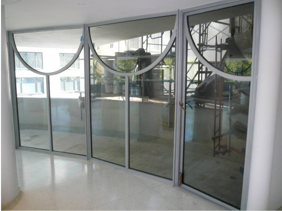
Fig. 7: The new windows replicated the existing in thermally broken steel.
