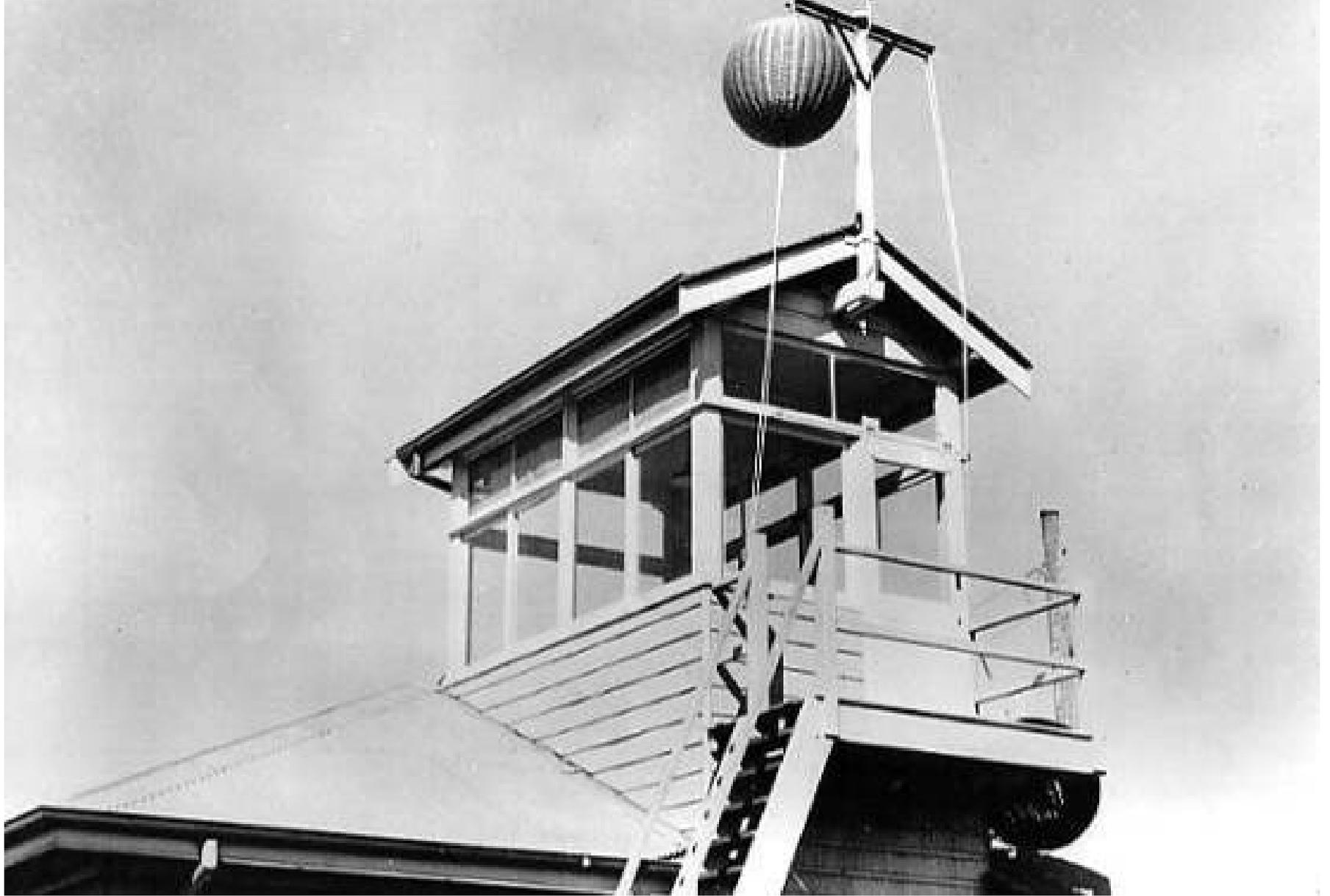
Sydney Mascot (NSW) c. 1936-7. The coloured cane sphere was a signalling device.
