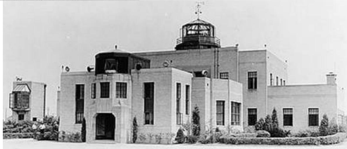
Cleveland Hopkins Airport (Ohio, USA) 1929. Integrated terminal and ATC control building surmounted by circular cabin
