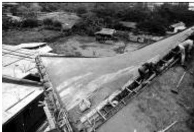
FIG 19 hyperbolic/parabolic roof under construction.
